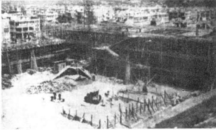
The New Building under Construction
